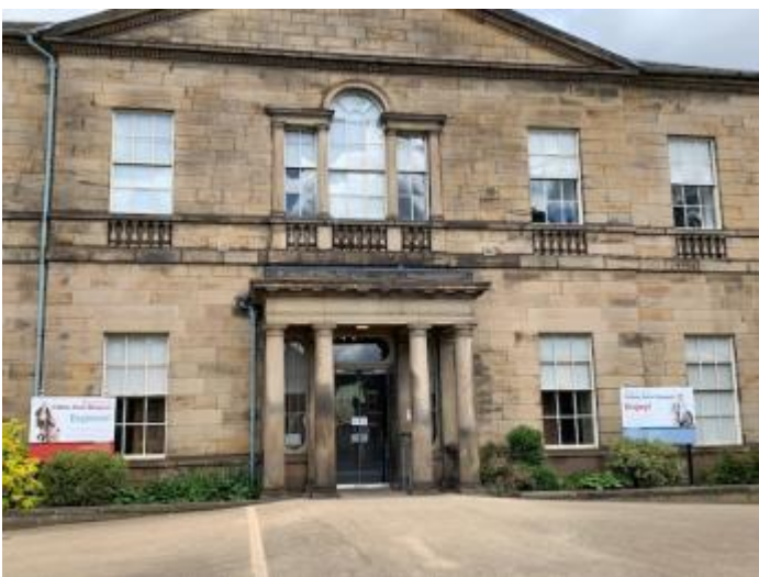
Image shows front entrance showing the slope and glass doors, these doors automatically open inwards
