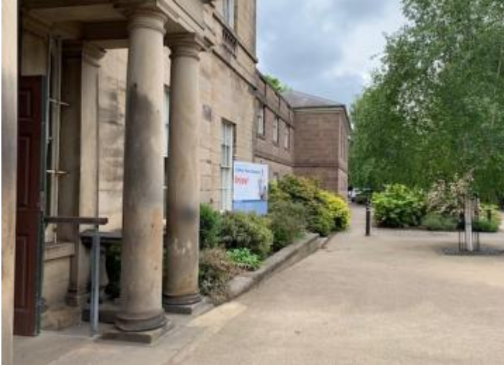
Image shows front entrance towards nearest Blue Badge bays
